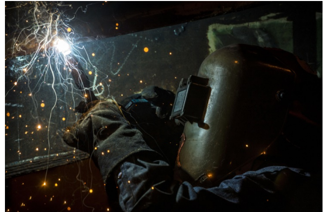
Mechanized and/or automated processes will reduce labor and improve quality during hull fabrication. Ingalls photo
